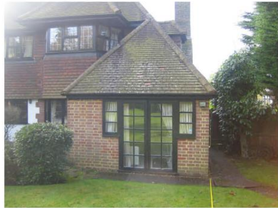
Existing Bricwork and Plain Roof Tile
